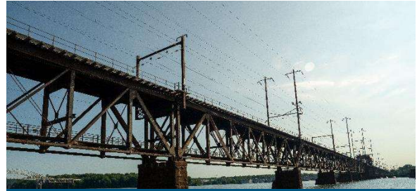
Susquehanna River Bridge
