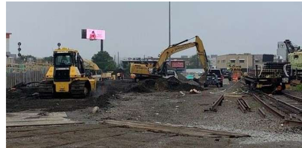
Southampton Yard ($136M)
