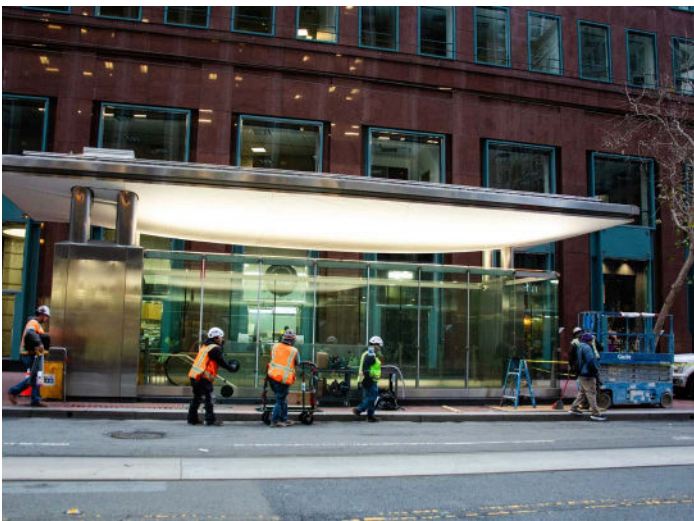
A new canopy being installed at an entrance to Embarcadero Station.
