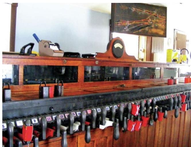
The 80-lever G pistol-grip electric interlocking machine was housed in a large wooden console. A track model board above the console showed the 80 switch locations on each of the railroad tracks.
