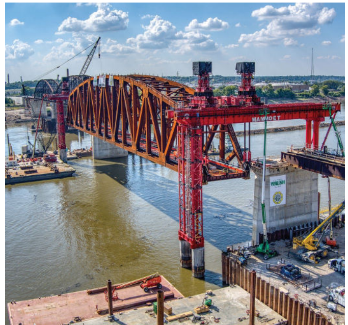
One of the three new trusses being installed
