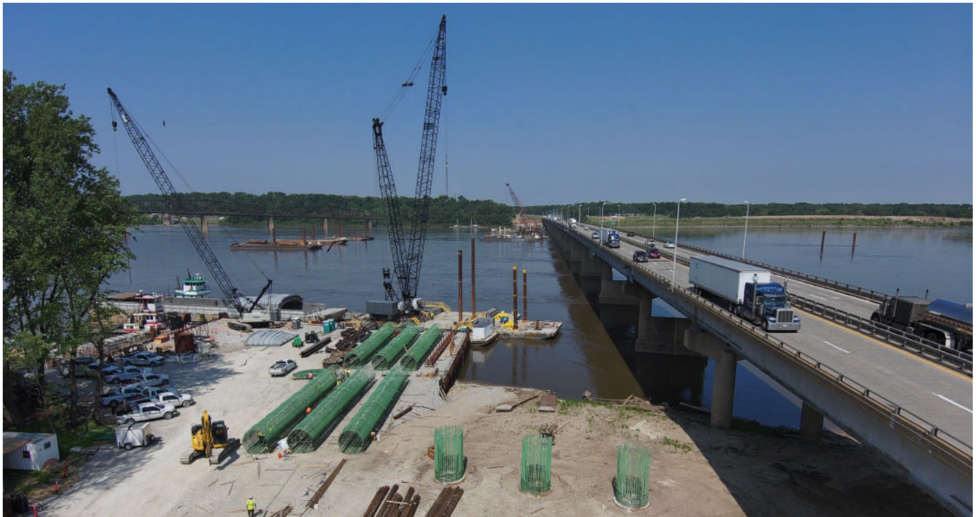
Chain of Rocks Canal bridge replacement
