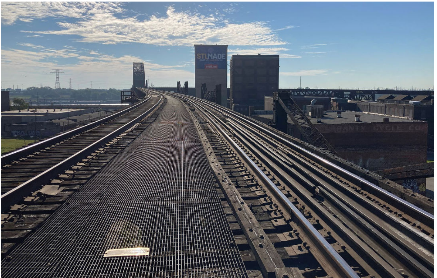
MacArthur Bridge just south of downtown St. Louis
