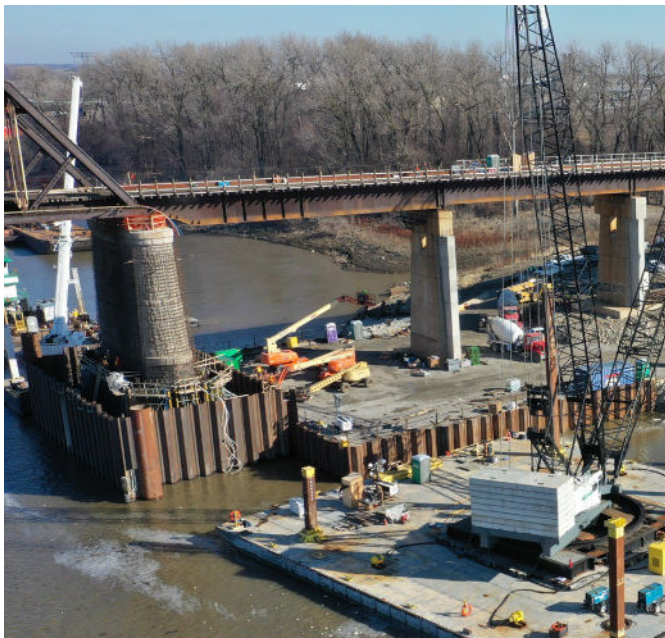
Constructing the bridge pilings
