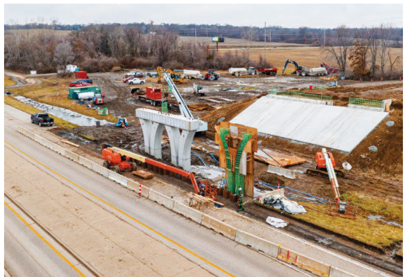
Progress on the new 5.5-mile MetroLink extension
