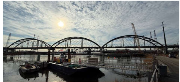
Portal North Bridge
