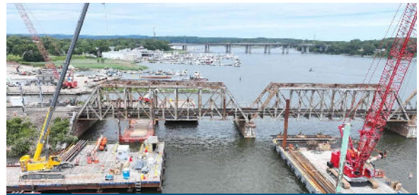
Connecticut River Bridge
