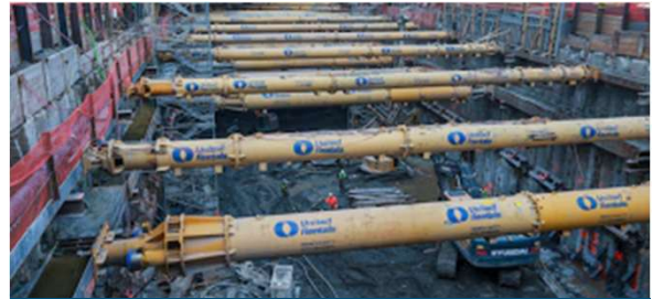
Hudson Tunnel Project
