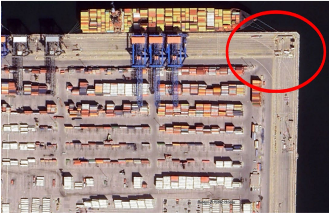
Figure 3.6.3: Berth 30A/31 Crane Conflict 24
