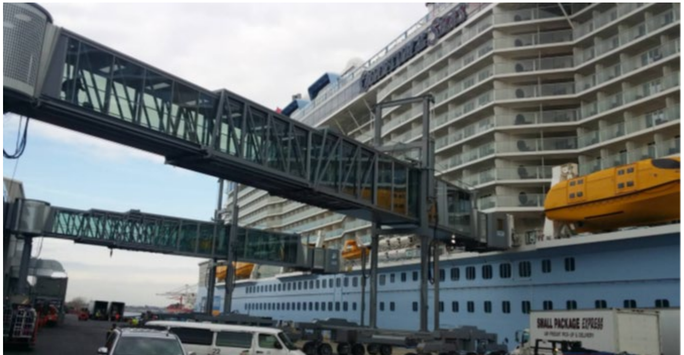
Figure 3.5.3: Example of Large-Vessel Gangway Service Range Needs 16
