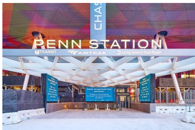
Caption: Amtrak unveiled its new, modern, and improved 7th Avenue and 32nd Street station entrance in November 2023, which reflects the types of improvements that will be advanced as part of the station transformation.
