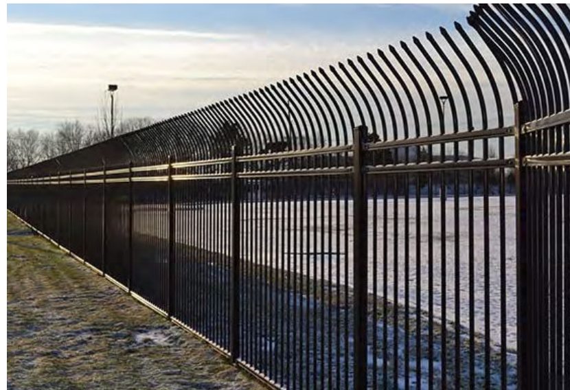
Figure 35. Security fencing Credit: MBTA
