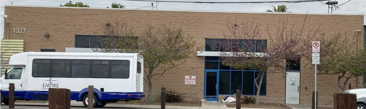
Figure 3 1327 W 12th Street, south elevation, view north (ERP 2025)
