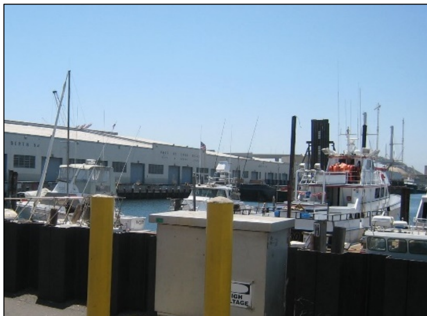
Figure 5. Transit Shed north façade facing south
