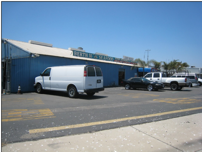
Figure 6. Berth 55 Fish Market and Seafood Deli east façade facing west
