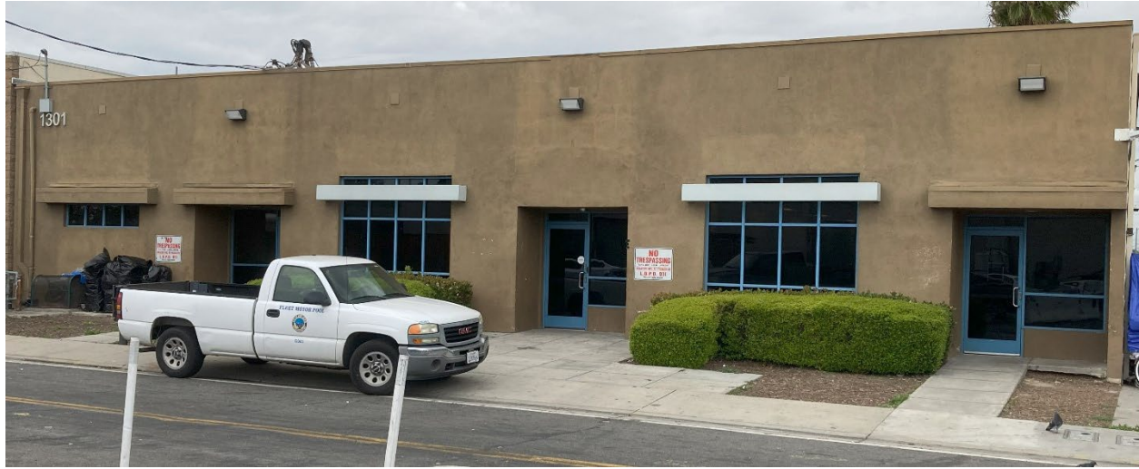
Figure 2 1301 W 12th Street, south elevation, view north (ERP 2025)
