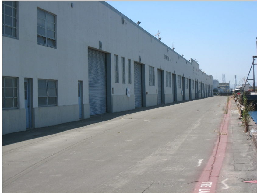
Figure 4. Transit Shed north façade facing south
