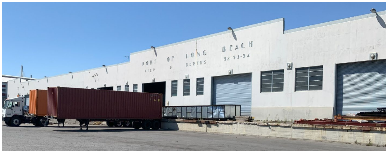
Figure 5 Transit Shed at Berths D52-D54, south elevation, view northwest (ERP 2024)
