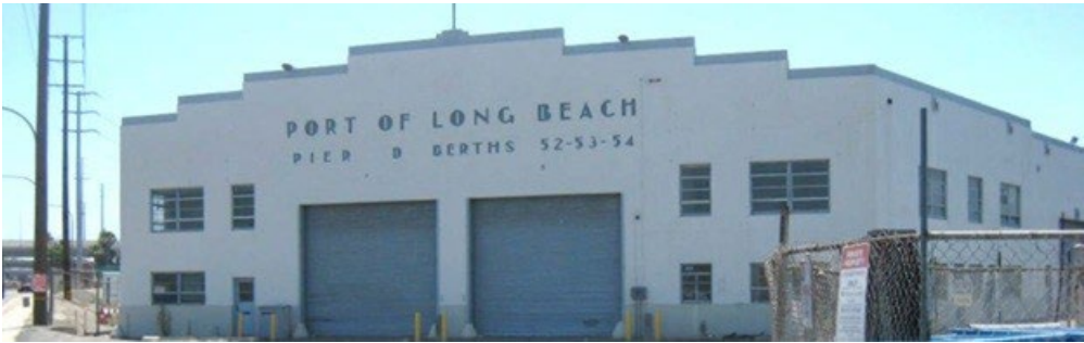
Figure 4 Transit Shed at Berths 52-54, primary (northeast) elevation, view southwest (ICF 2019)
