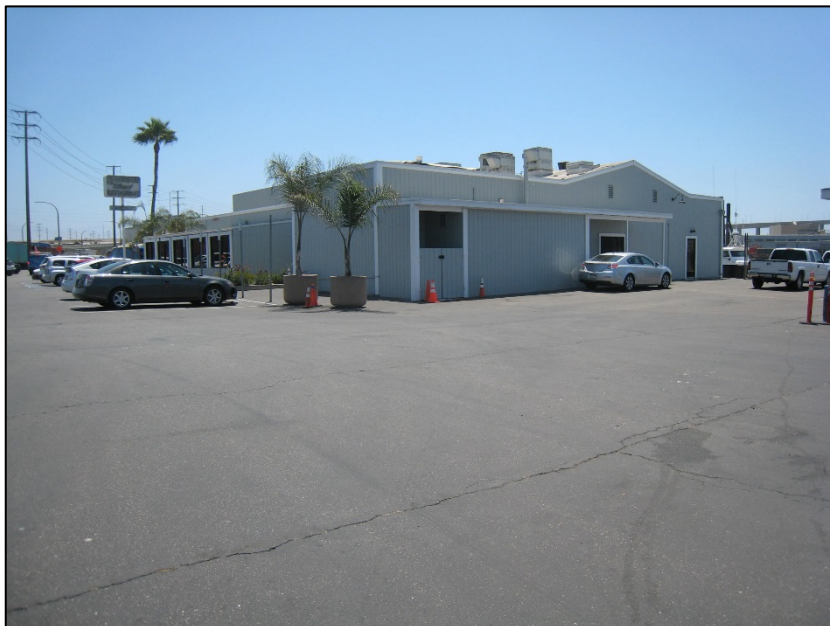
Figure 7. Queen's Wharf Restaurant and Bar north and east façades facing south
