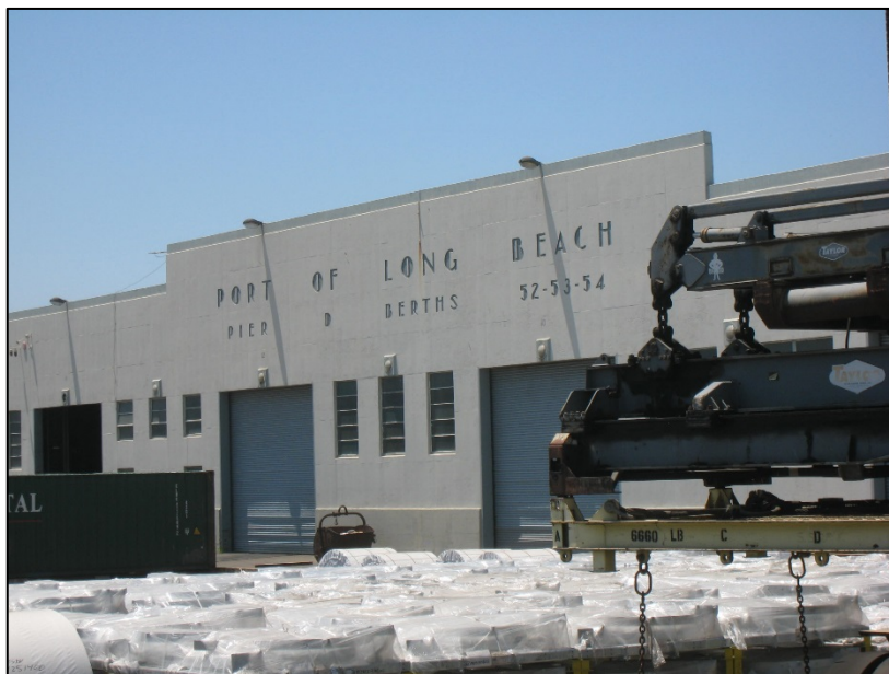
Figure 3. Transit Shed southeast façade facing north
