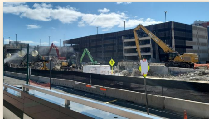
A photo of the old STC parking garage demolition from August 2024.
