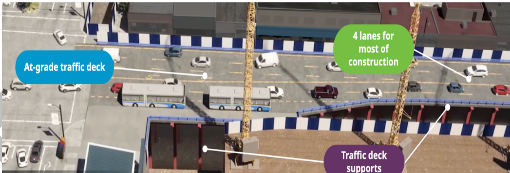
Figure 8 - Traffic Decking for Broadway Subway Project, Vancouver, CA
