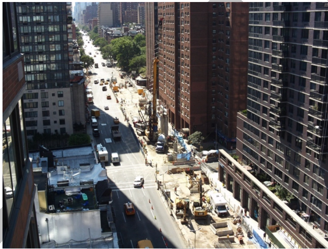
Figure 5 - 96th Street Station slurry wall construction, 2nd Avenue Subway, New York
