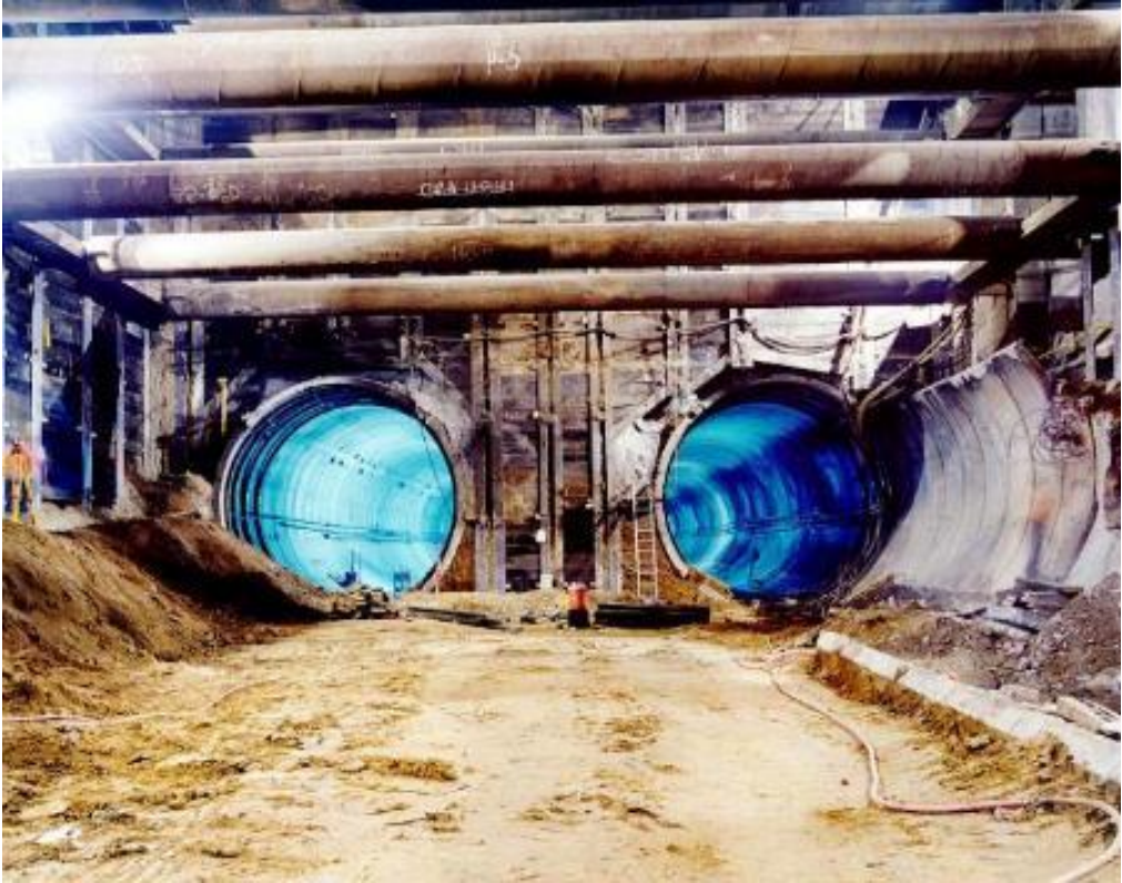
Figure 1-9 Twin Bore Tunnel with Excavation Support
