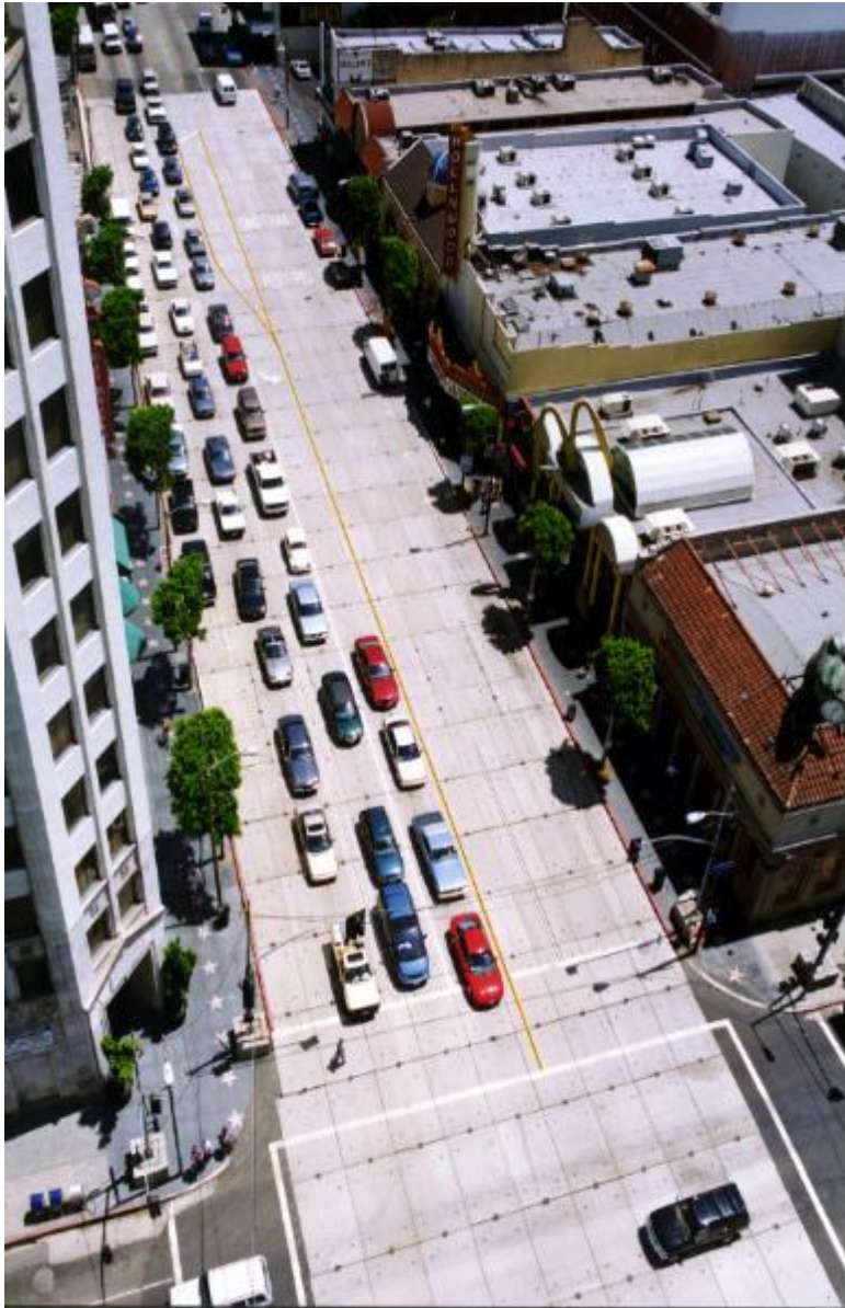
Figure 1-10 Typical Deck Covering over Excavation
