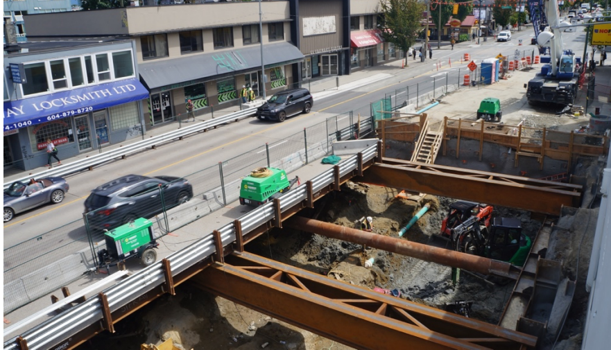
Figure 9 - Broadway subway construction near Yukon Street, Vancouver
