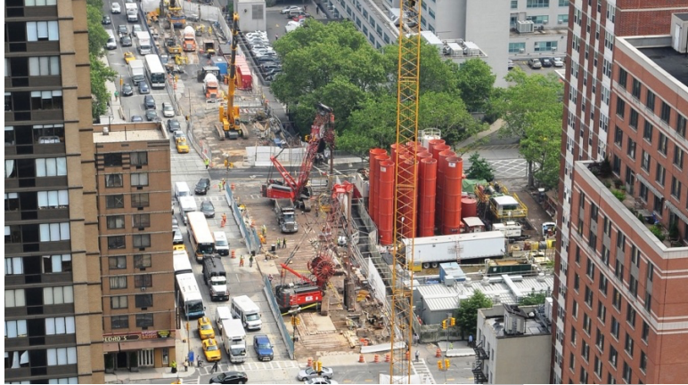
Figure 4 - 96th Street Station staging area, 2nd Avenue Subway, New York
