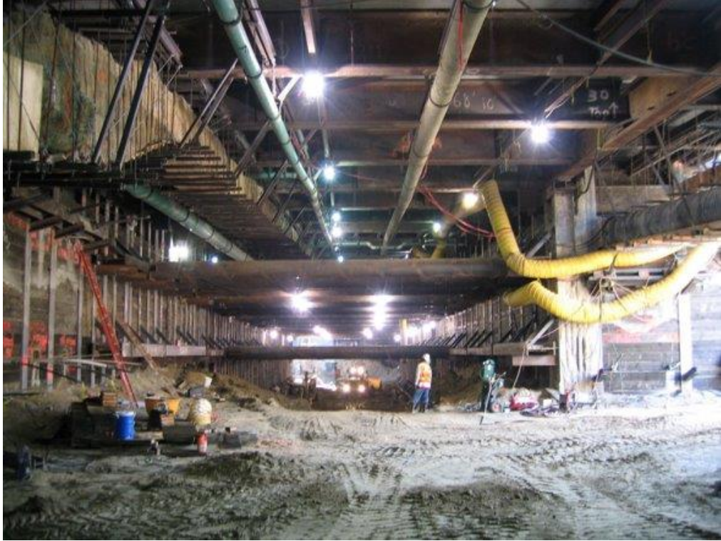
Figure 1-8 Cut and Cover Underground Station Construction
