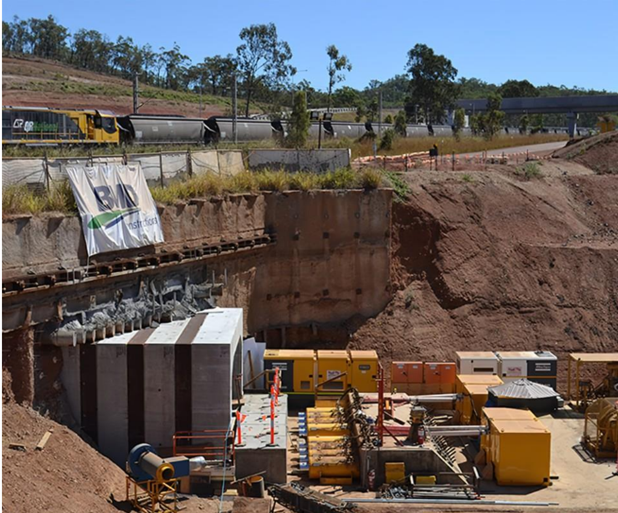
Figure 2-4 Construction of Jacked Box under Operating Railroad Tracks
