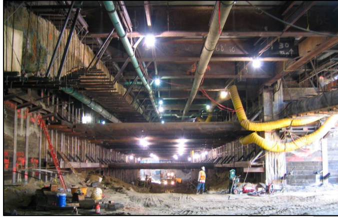
Figure 14 – Support of utilities by decking beams (LA Metro)
