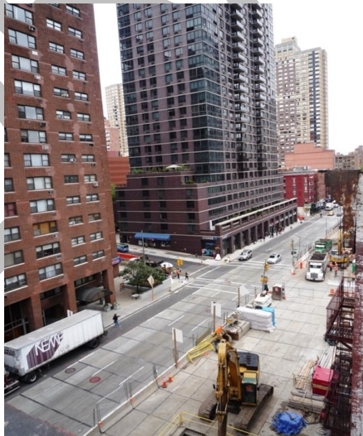
Figure 6 - 96th Street Station Street Decking, 2nd Avenue Subway, New York
