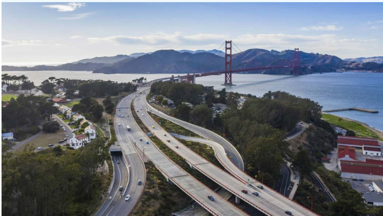
Presidio Parkway in San Francisco (SOURCE BAY AREA COUNCIL)
