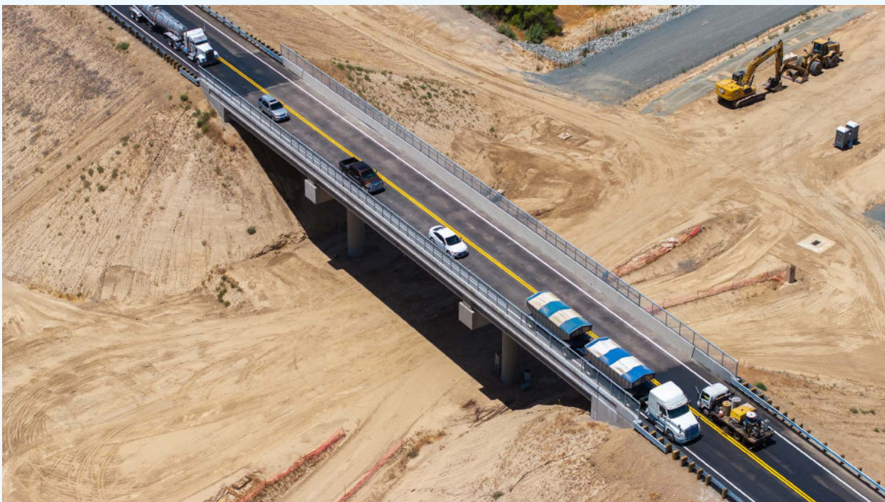
The Avenue 56 Grade Separation in Tulare County was completed in June 2025 and spans a length of 219 feet.
