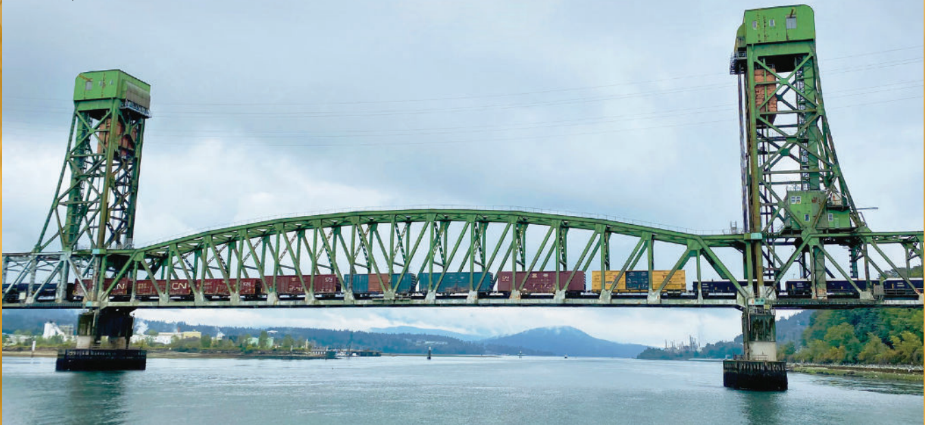
Second Narrows Bridge Vancouver, BC
