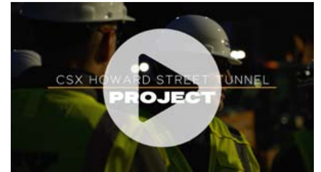
Watch a brief video of the Howard Street Tunnel construction
