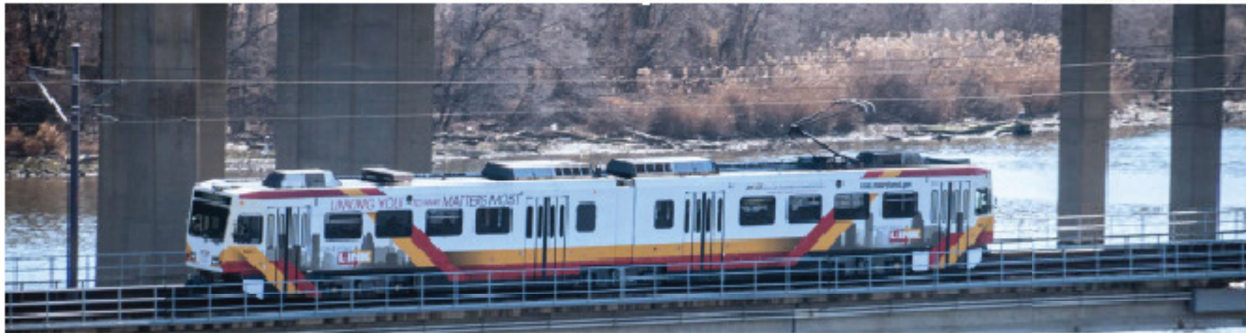
Light Rail Southern Track Maintenance
