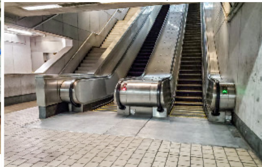
Penn-North Escalator Replacement
