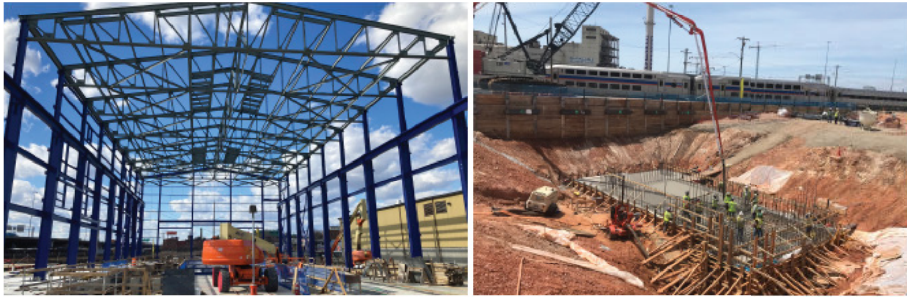
New Marc Train Riverside Heavy Maintenance Building
