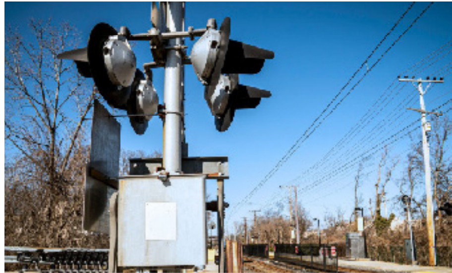
Light Rail North End Signal Power System Replacement
