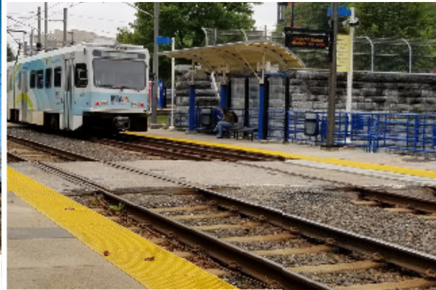
Light Rail Catenary System Rehabilitation
