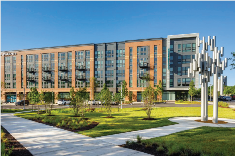
College Park—Atworth (Gilbane), 2024 451 units (100% affordable)
