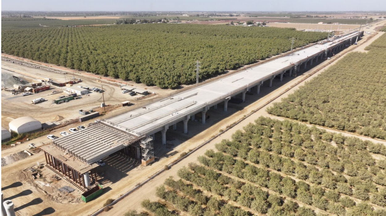
The Hanford Viaduct in Kings, California
