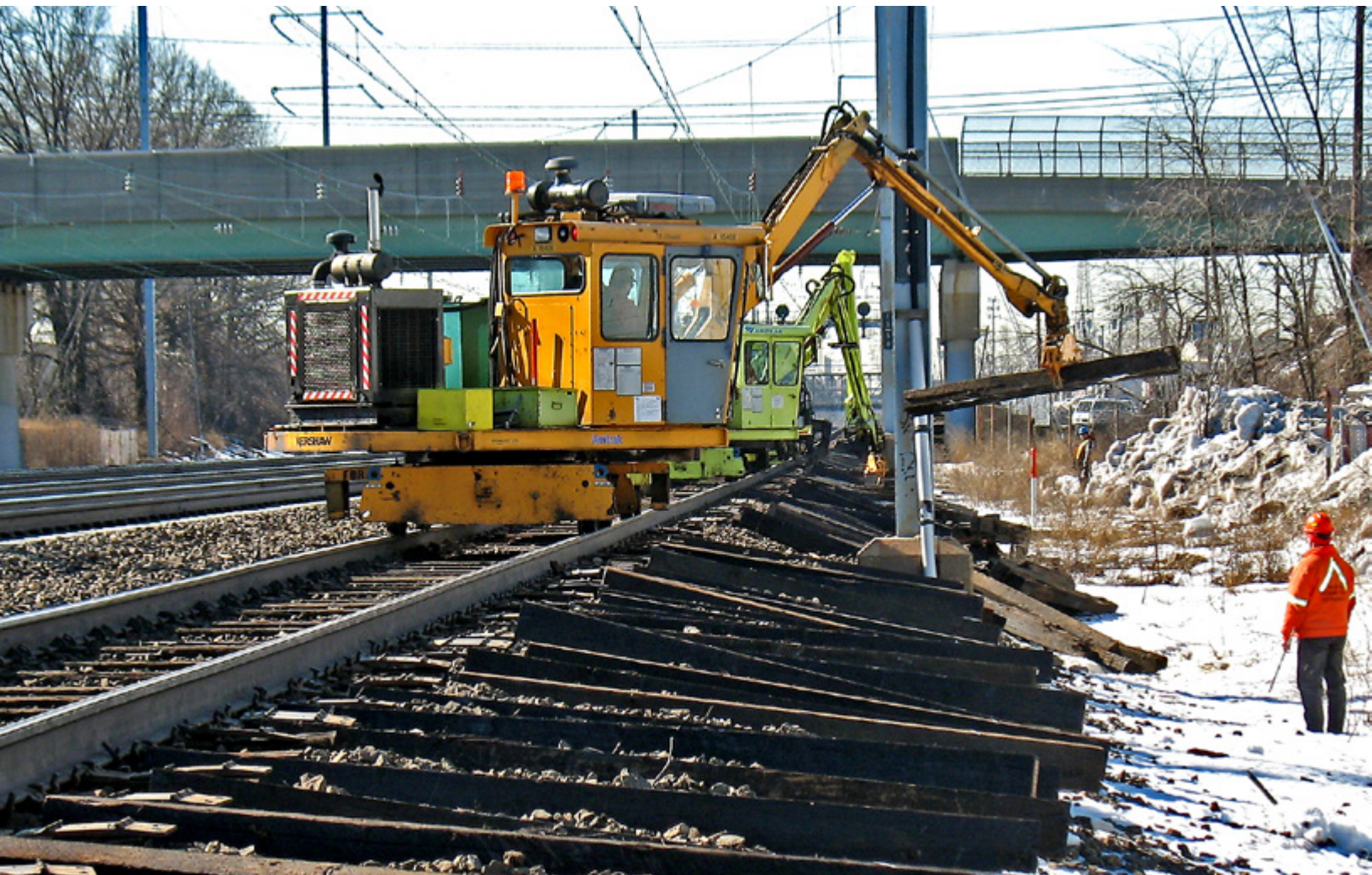
Above: Track tie renewal work near Elizabeth, New Jersey
