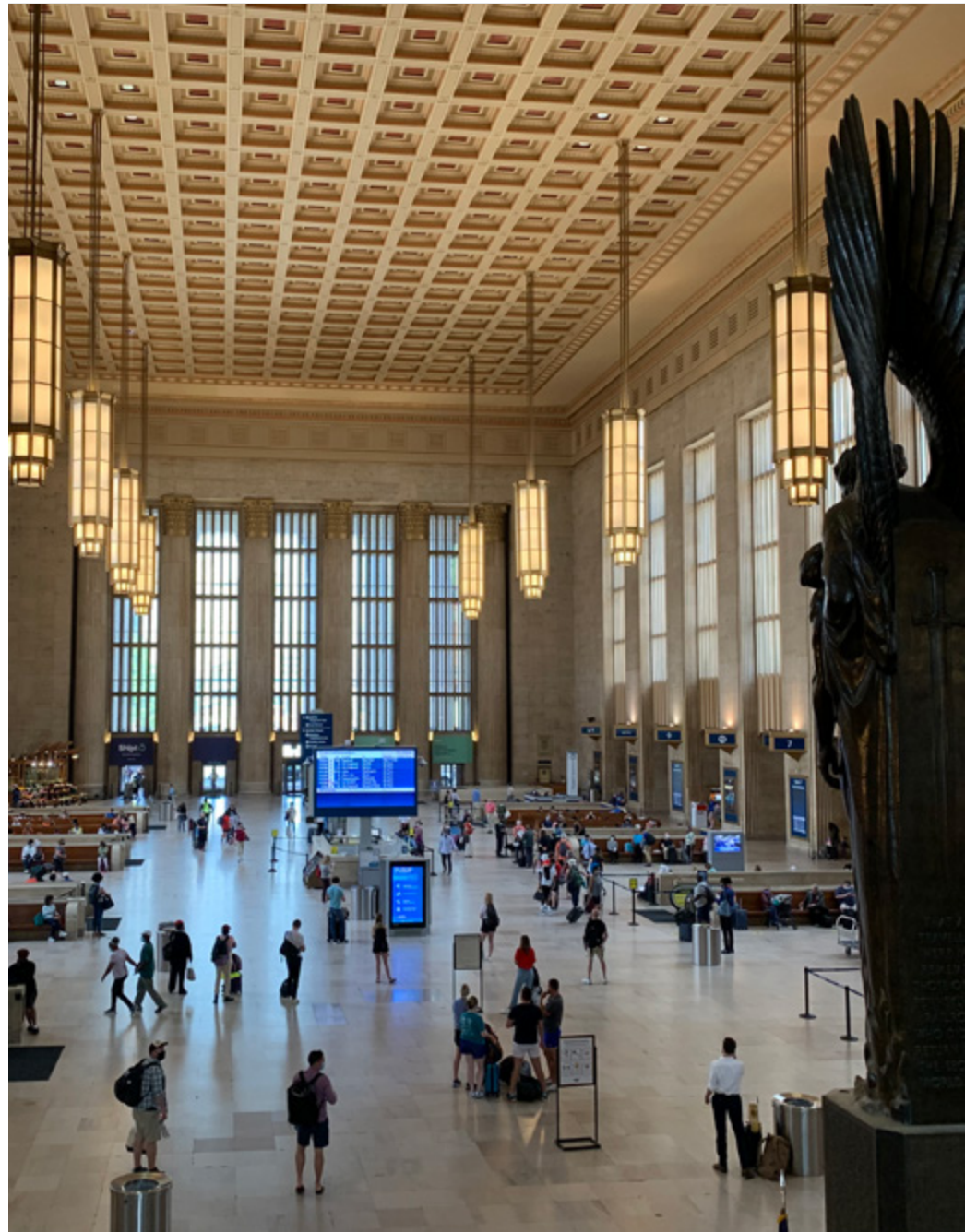
Above: Philadelphia's William H. Gray III 30th Street Station's renovation is being completed in phases to maintain Amtrak operations. The full renovation is anticipated to be complete by the end of 2027.
