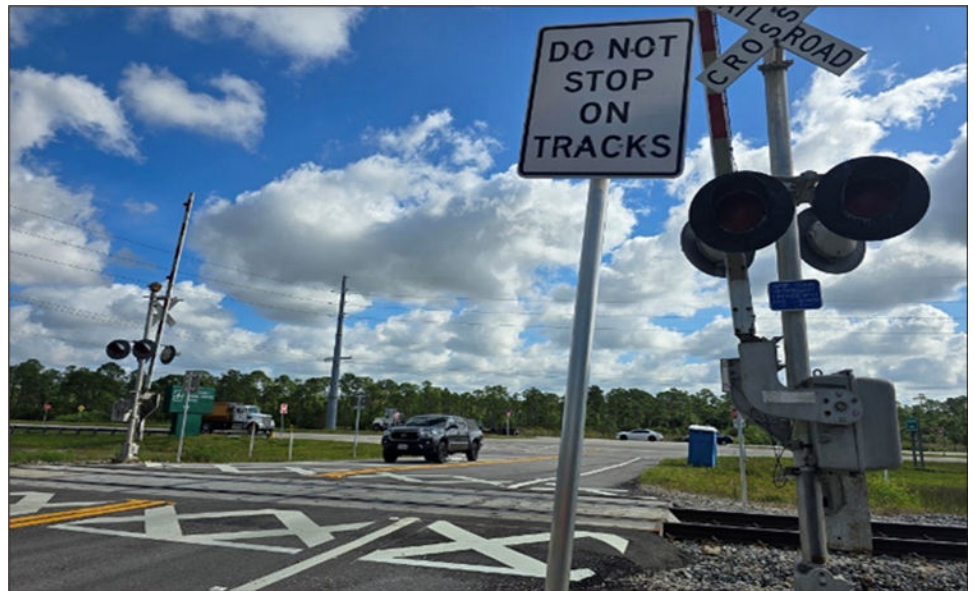
Figure 11: Completed Railway-Highway Crossings Program Project in Palm Beach County, Florida, That Upgraded Signals, Gates, and Lights and Added Dynamic Envelope Markings Near the Grade Crossing
