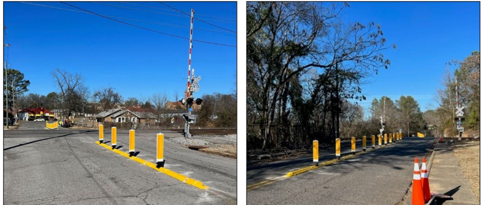
Figure 9: Completed Railway-Highway Crossing Program Project in Alabama That Installed Delineators at Two Different Grade Crossings
