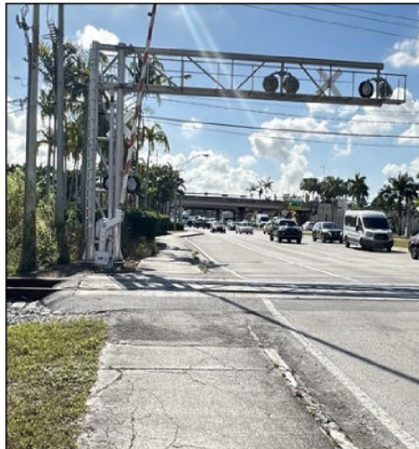
Grade crossing without a pedestrian gate. The state plans to install an additional gate arm for pedestrians with Railway-Highway Crossings Program funding. (Doral, Florida).
