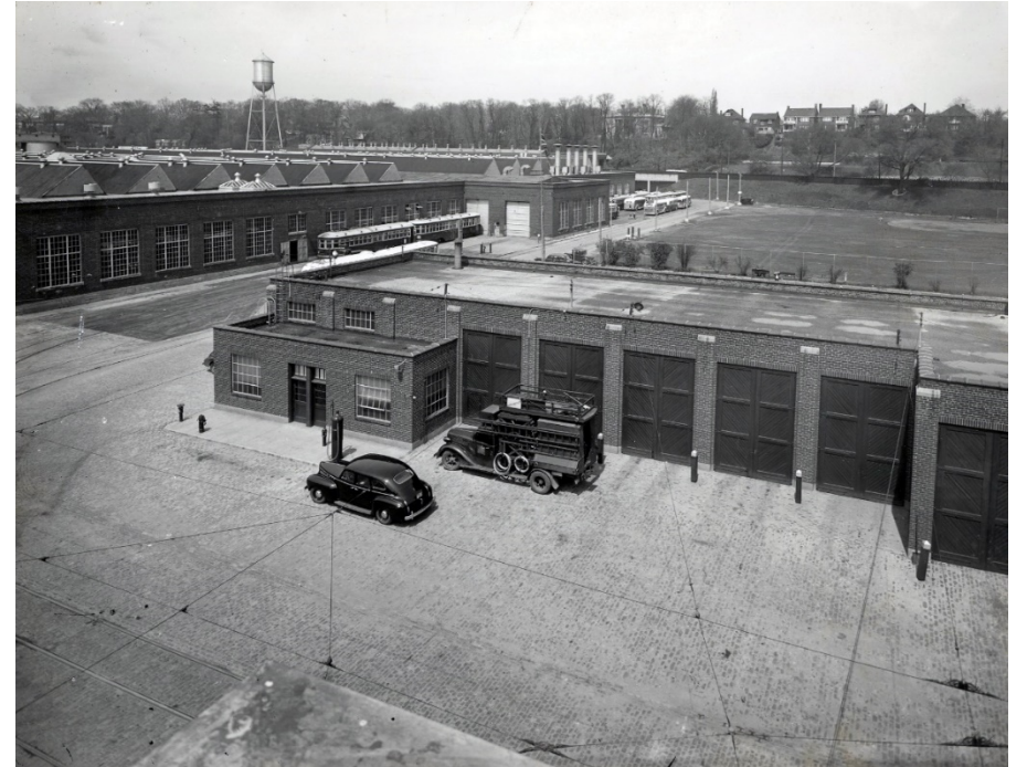
Hillcrest Complex looking north towards Davenport Road (1944).
