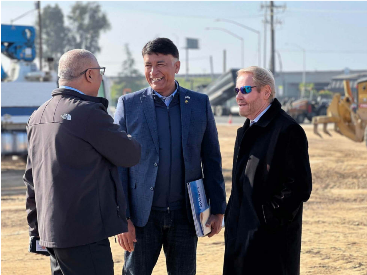
Photo: CEO Ian Choudri (center) with Chair Tom Richards (right) at the groundbreaking of the McKinley Avenue and Golden State Boulevard Grade Separation Project
