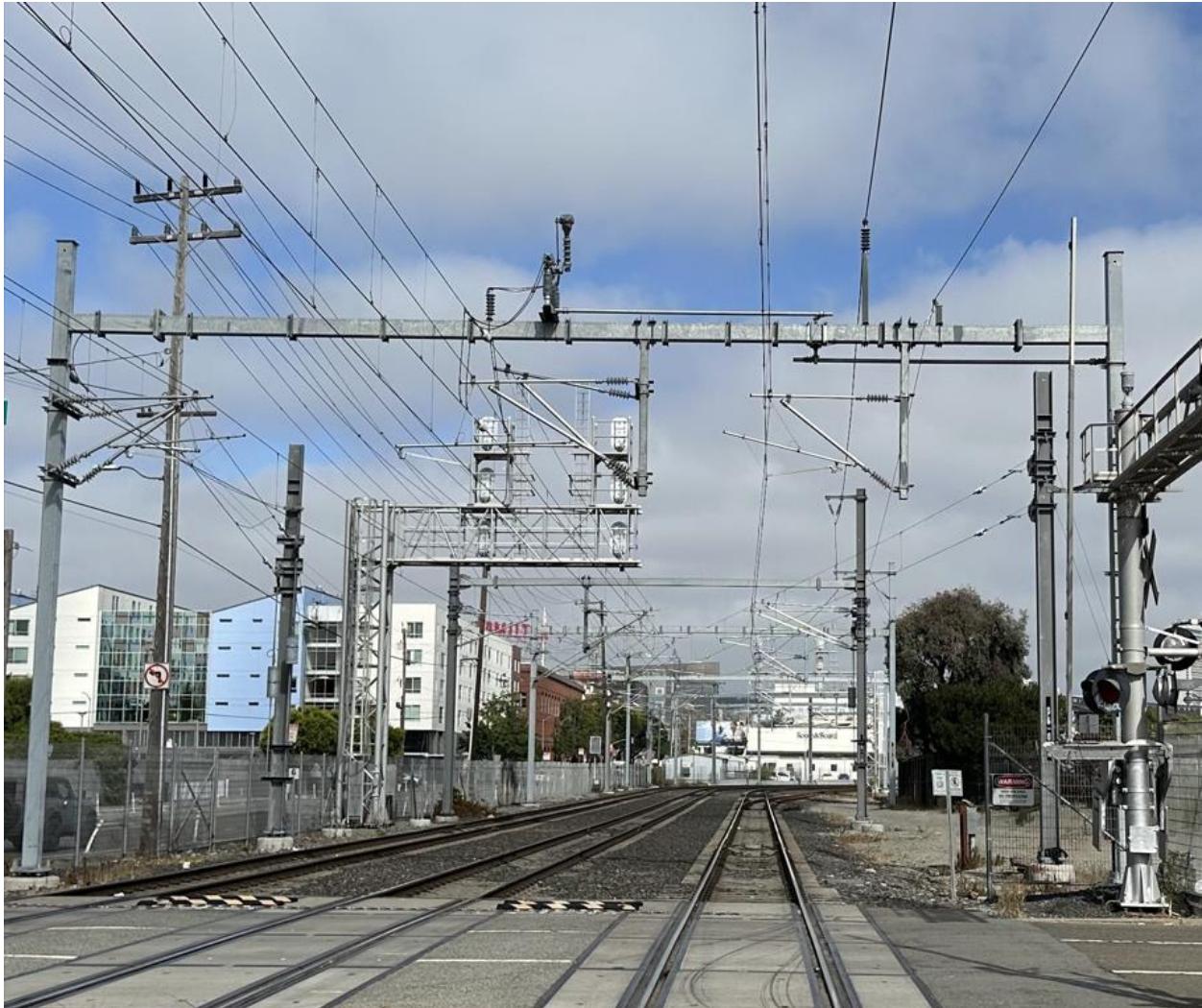
Figure 6: Example of Portal Construction.
