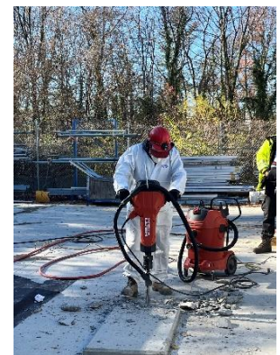
Electric jackhammer demonstration
