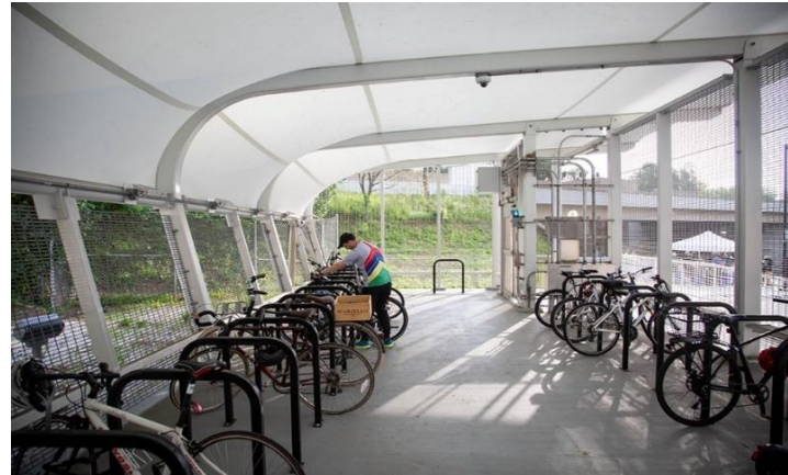
East Falls Church Metrorail Station Bike & Ride
