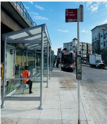
Rhode Island Ave-Brentwood Station Bus Shelter
