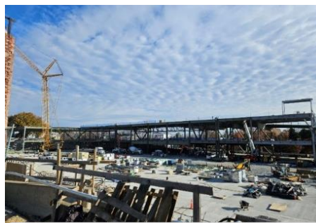
Construction underway at Northern Bus Garage
