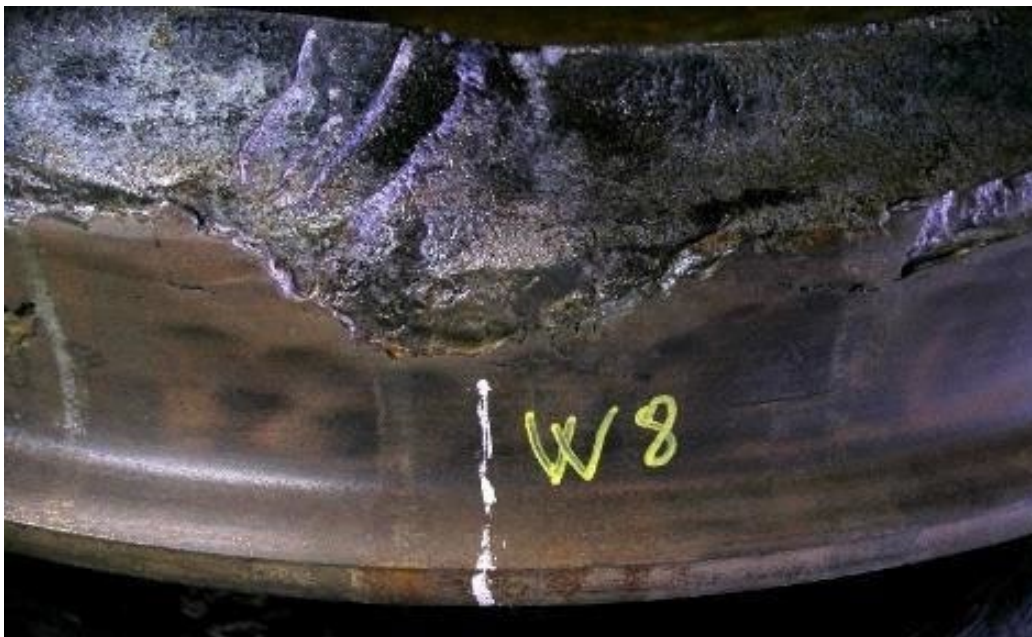
Figure 3. A VSR failure with deformed steel and purple coloration exhibiting high temperature exposure
