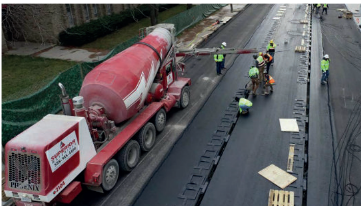
Workers filling trench and placing coils prior to paving on 14th Street
