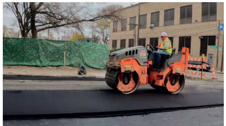
Roller compacting new pavement on 14th Street
