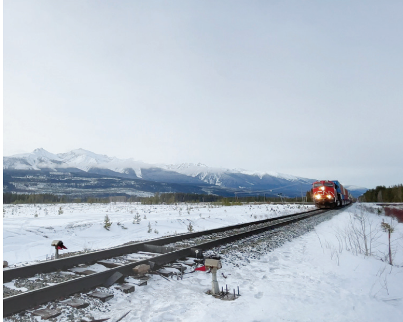
Wayside detectors in foreground stand ready to inspect approaching CN train in Blue River, BC.
