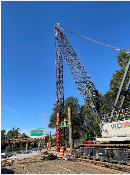
Test pile driving in fall 2023.
