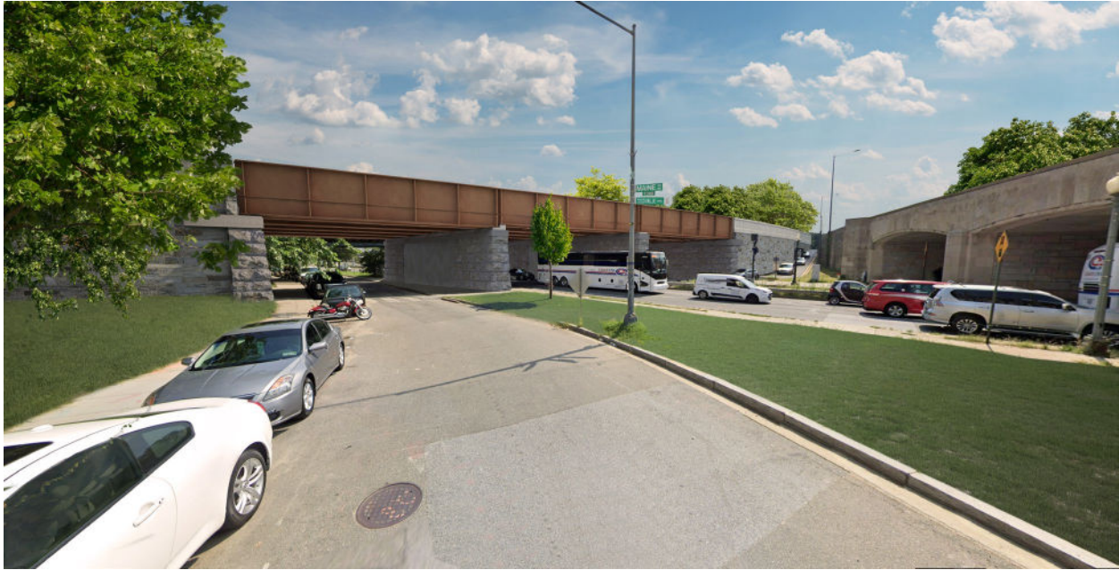
The replacement of the two-track Maine Avenue SW rail bridge in Washington, DC with a four-track bridge is one of the components of the Long Bridge Project's North Package.
