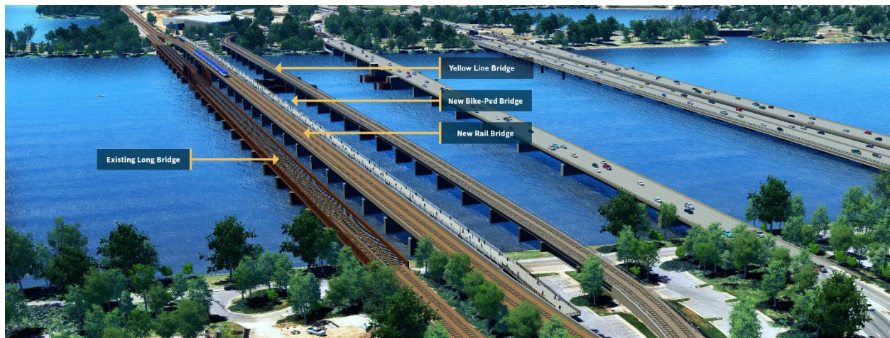
A rendering of the Long Bridge Project section over the Potomac River highlighting the new rail bridge and new bicycle-pedestrian bridge.
