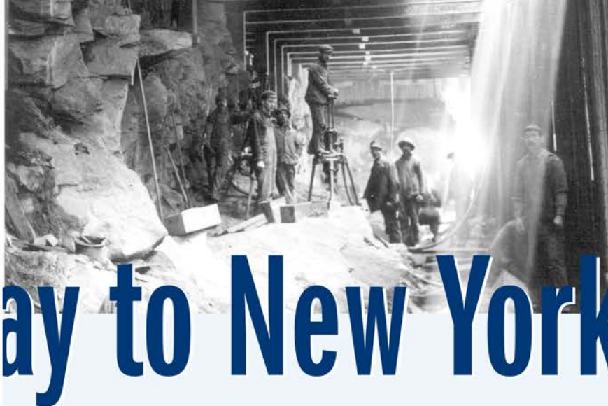
Far left: Building is under way on the Lexington Avenue Line south of City Hall Station. (Park Row; 1902)
