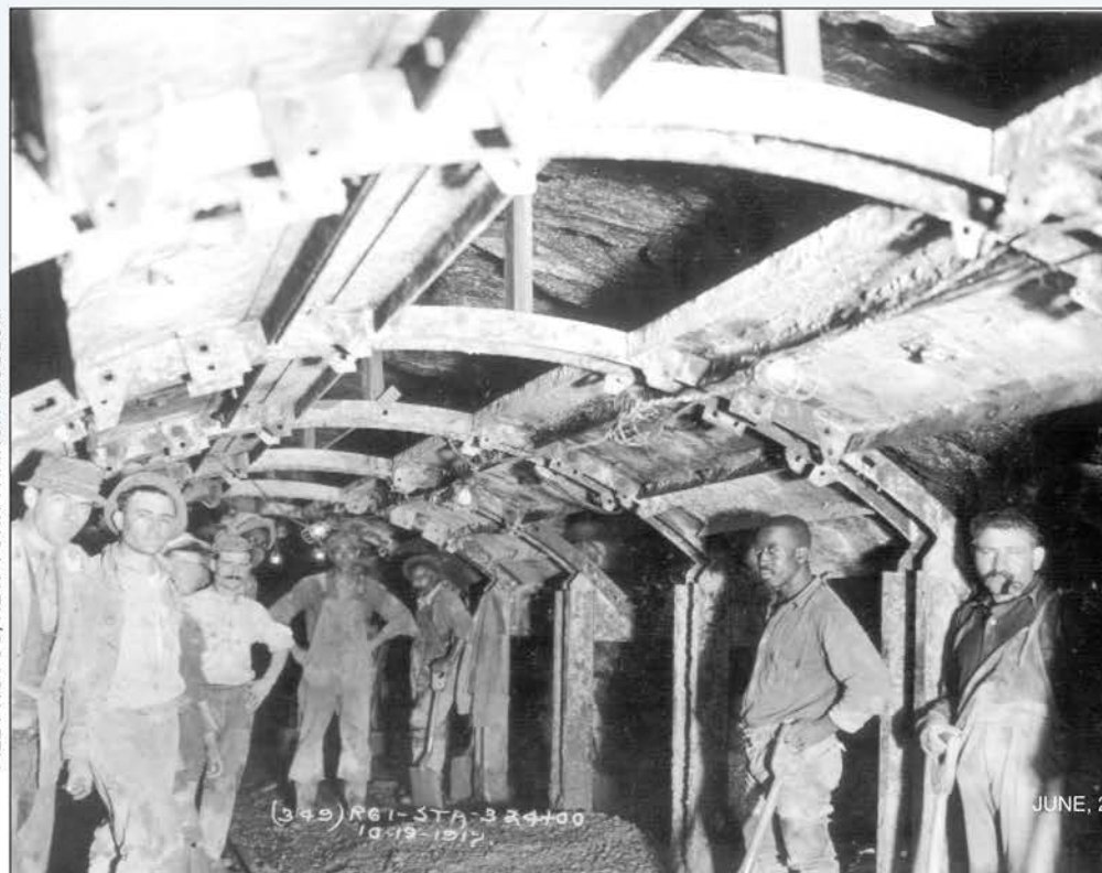
"Sand hogs" continue their work in the tunnel under Joralemon and Furman Streets. (60th Street Tunnel; 1919)
