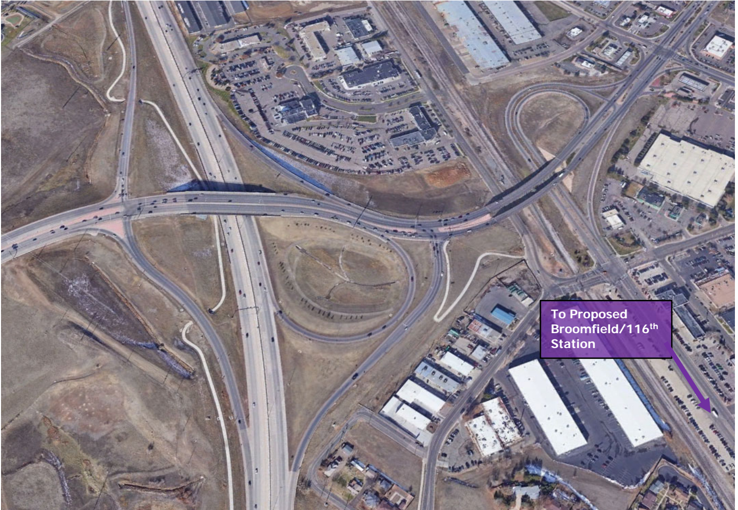
Figure 21: US 36 at Wadsworth Parkway/US 287 Interchange
